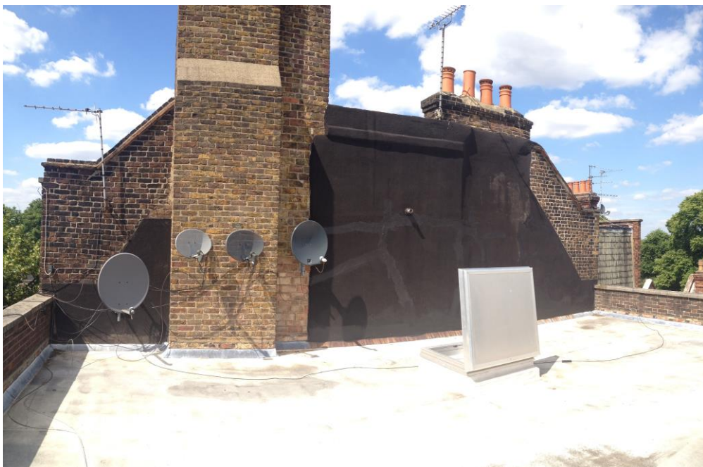
Image 2: View of neighbouring mansard roof
